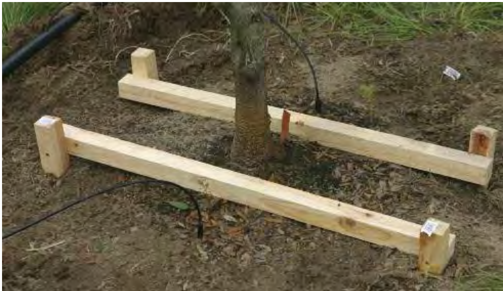
FIG. 19 BIODEGRADABLE ROOT ANCHOR USING UNTREATED TIMBER
